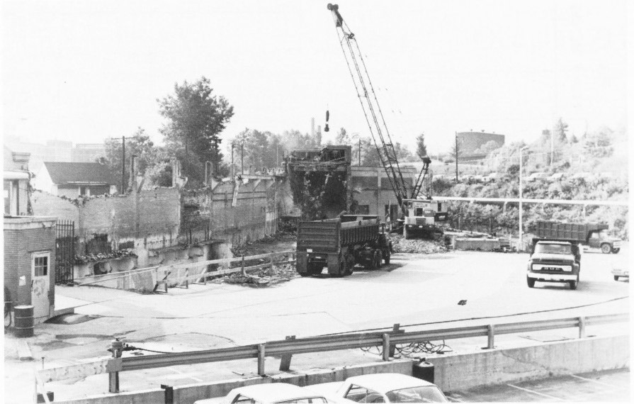
Oil House Makes Way for Waste Treatment Plant
